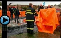
the use of a non-permeable membrane (supplied) is necessary to prevent seepage
